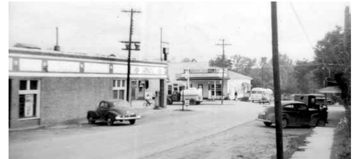
Looking South on 2nd Street to intersection with Highway 84 in downtown.
